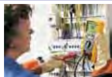
Insulation test at a distribution panel
